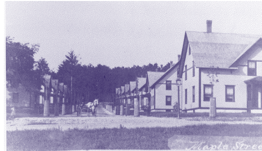
These houses for Whitin employees were built in 1889. Workers with higher status in the mill enjoyed larger, more attractive living quarters than those with lower rank. Eventually, the town contained more than a dozen clearly differentiated levels of housing.
