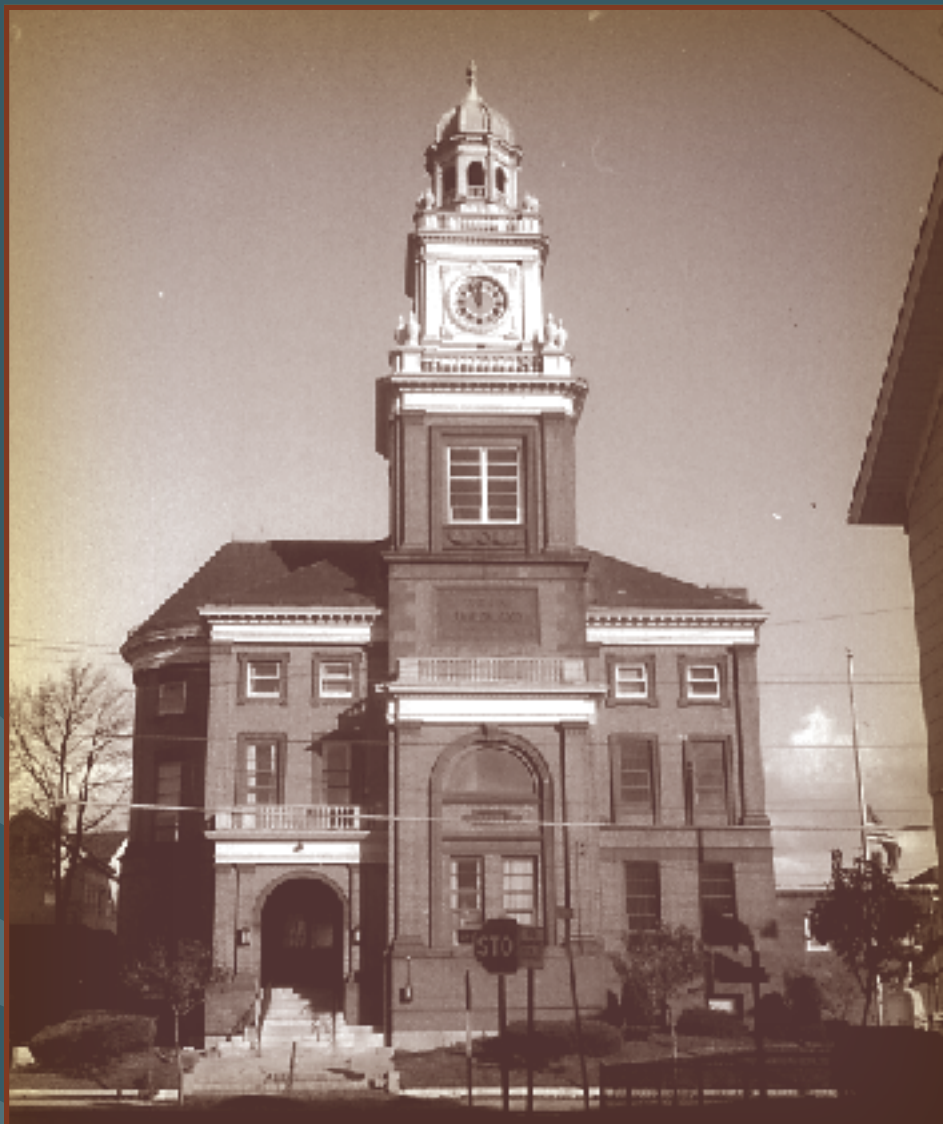
Cumberland Town Hall. Photo courtesy of Kevin Klyberg.
