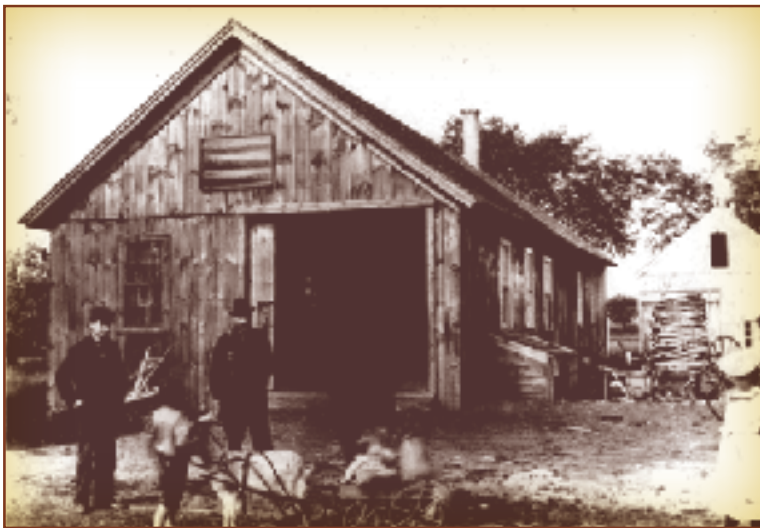
Despite the Center's bustling business, there was not enough blacksmith work to support both Daniel Dudley's shop and that of his neighbor, Milton Sherman. Within a few years, Dudley sold out to Sherman, who built an addition and a building for lumber. The Sherman blacksmith and wheelwright shop, shown here in 1893, is currently a working shop, run by the Sutton Historical Society.
