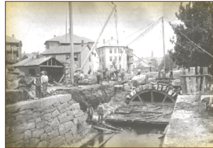
When the Blackstone Canal Company folded, parts of the abandoned trench deteriorated into rank open sewers. During the 1890s, they were sensibly integrated into Worcester’s underground waste water system. Dressed granite blocks from the 13-foot walls of the 82-foot long locks were sold and carted away to become parts of new buildings. During deep excavations, the city’s highway department even now sometimes uncovers the canal.
